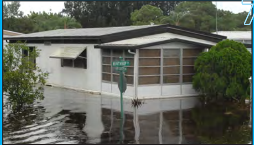
Major: 3," standing water, Mobile Home (MH)
