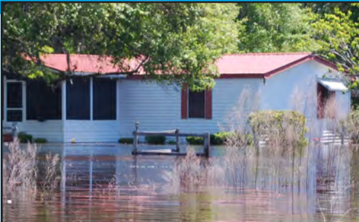
Minor: 10," standing water, Single Family (SF)
