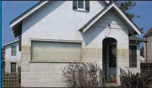
Destroyed: 5,' standing water, Single Family (SF)
